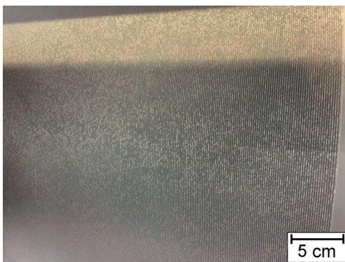
Fig.11. A corroded sink roll.
